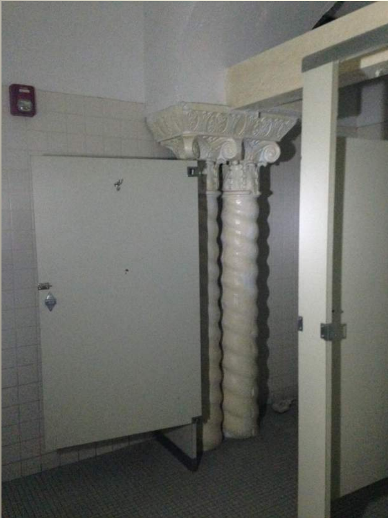
Solomonic Columns now located in the restroom. Due to the change in floor slope, the bases are now below the floor slab.
