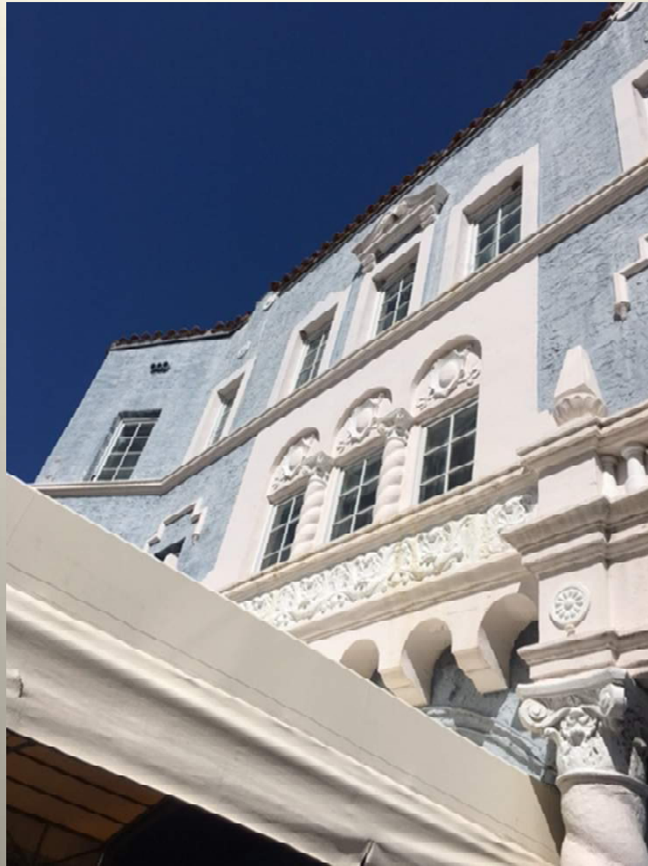
Current Playhouse Exterior showing detail at the Front Elevation
